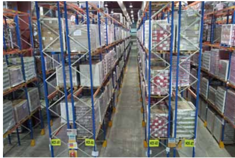
The warehouse at HRDC is one of the largest structures in Afghanistan
